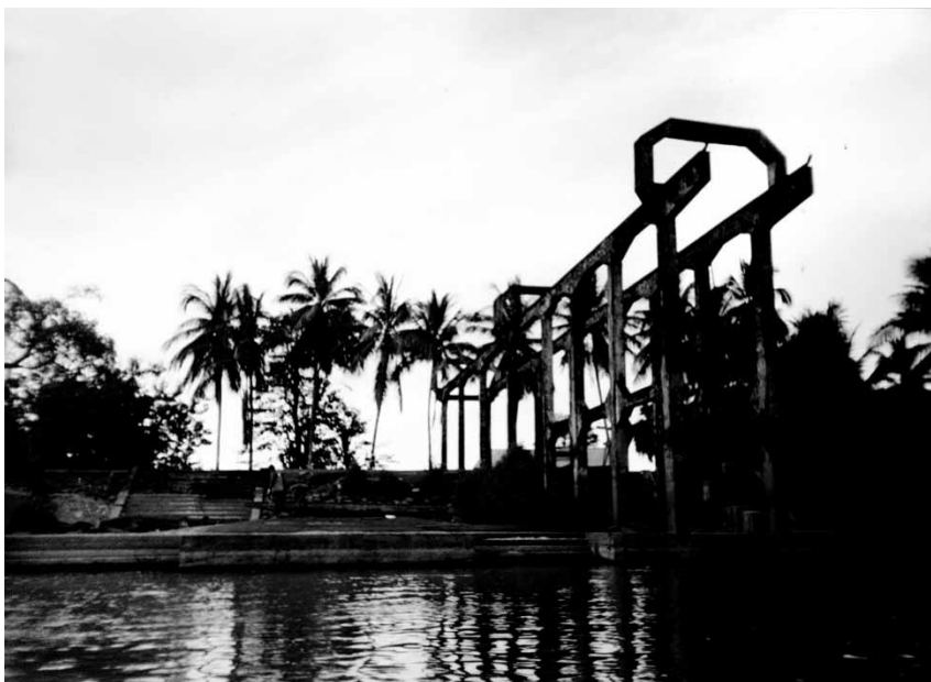
Plate 3 Rail-to-boat gantry above the Khon Falls
