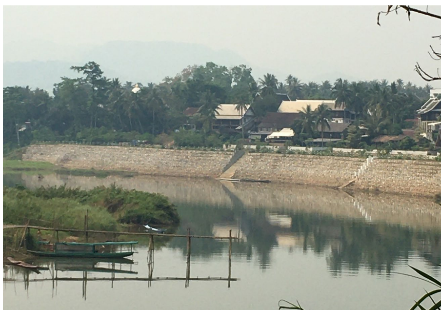
View of the riverbank protection work (©N.HAYASHI2022)
