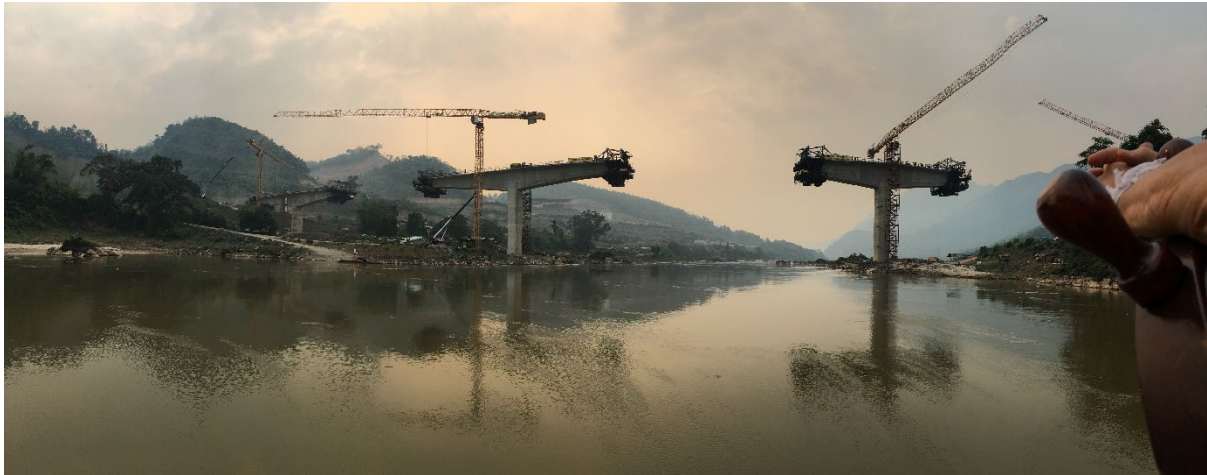
Hydropower construction preparatory site, as seen on 7 April 2022 (©N.HAYASHI2022)
