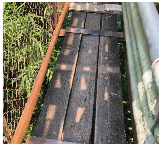
Pedestrian pathway of the bridge ©UNESCO N. Hayashi 2022
