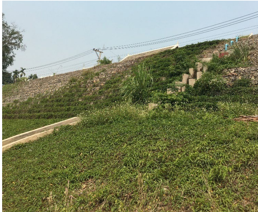
Segment of riverbank protection by gabions and RipRap, with vegetation ©N.HAYASHI2022
