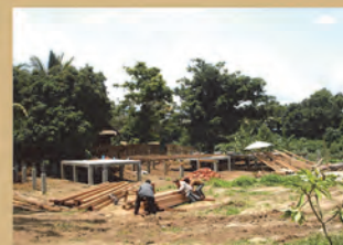
Demolition of construction
