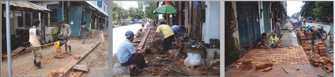
Construction and Restoration Works
