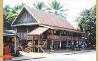
Picture after restoration
