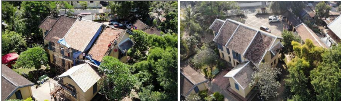
Replacing roof material
