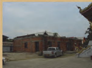
Demolition for improvement
