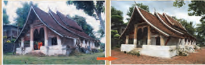
Before restoration After restoration
